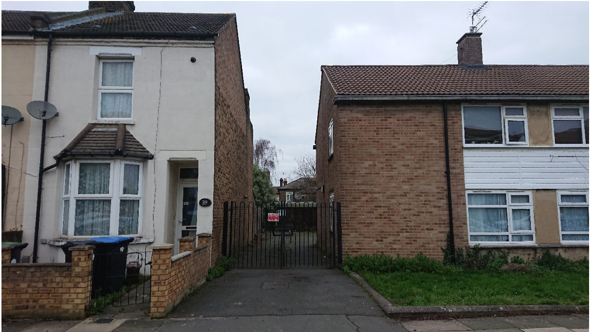
Figure 5: West-facing flank windows on the other end of the residential block (Nos. 23 – 37).
