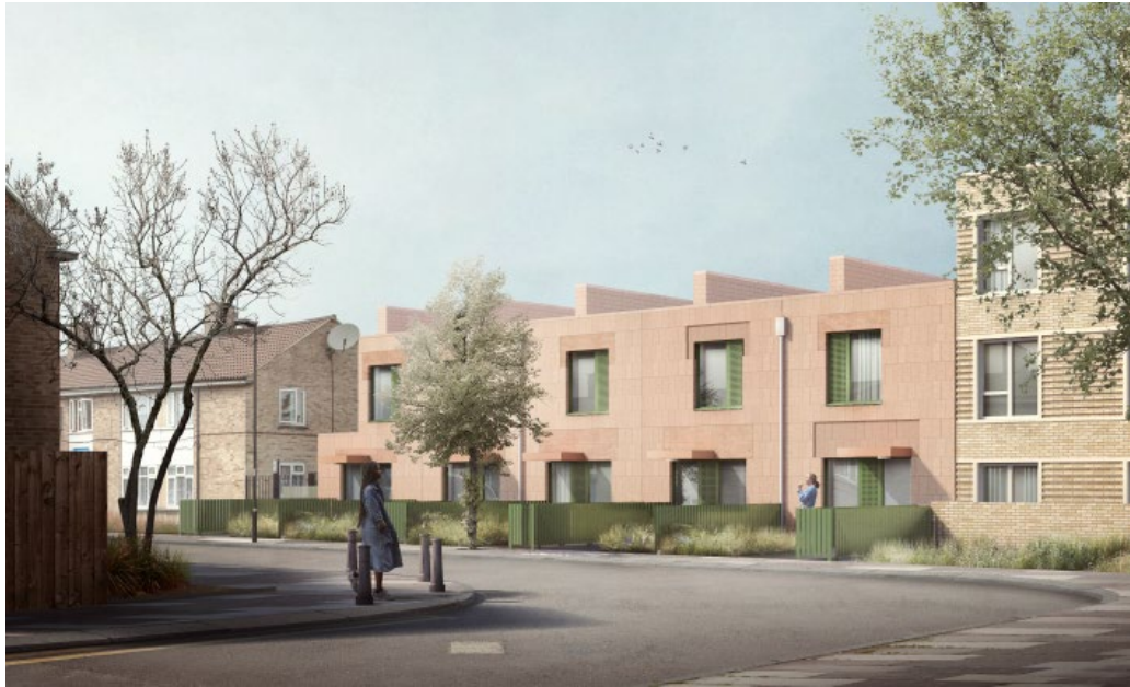
Figure 2: View facing Raynton Road at naked state
